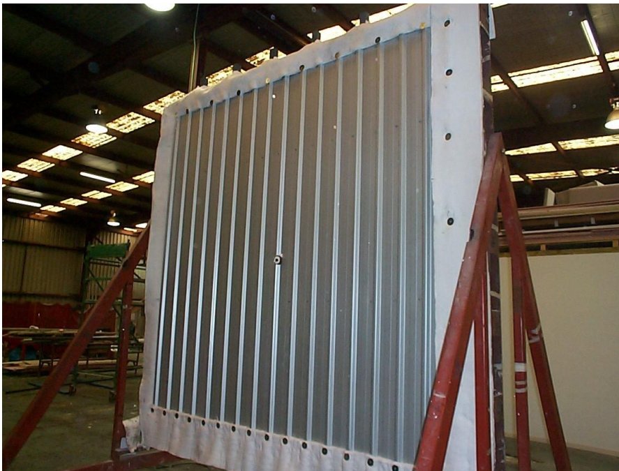
Figure 3 Exposed side of wall system
